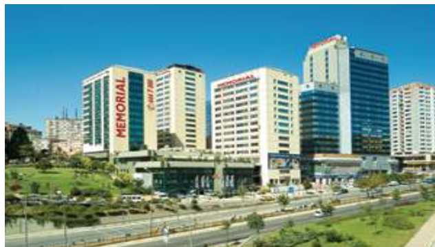
▲ Istanbul Memorial Hospital 전경
